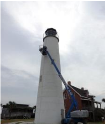
Hairline stucco cracks were dug out and filled.
