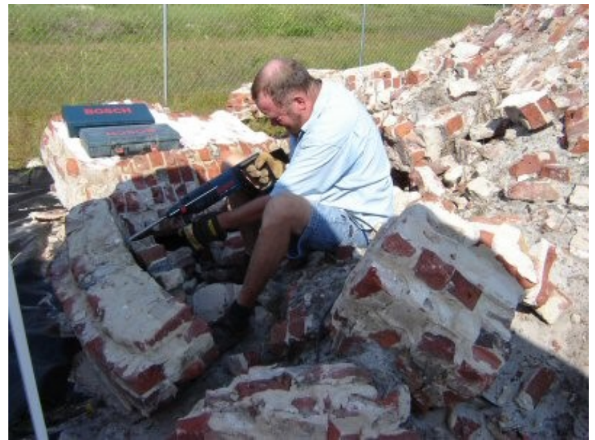
Dennis Barnell breaks smaller chunks of bricks from the large lighthouse pieces salvaged from Little St. George Island in Spring of 2006. Taken: 10/6/2006
