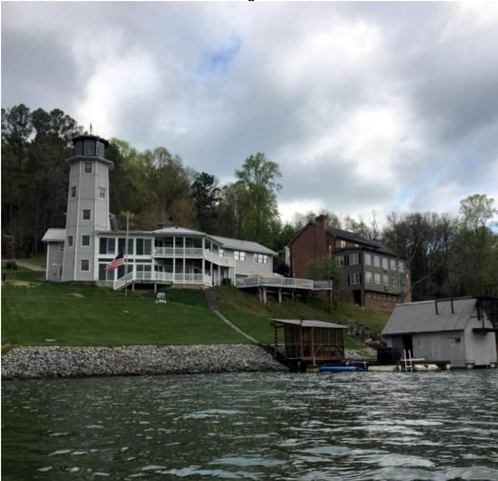
Completed Baie de Caracol Lighthouse
