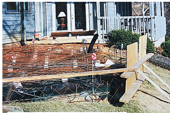
Foundation rebar
