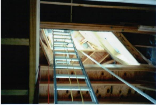
Ladder going up stair opening
