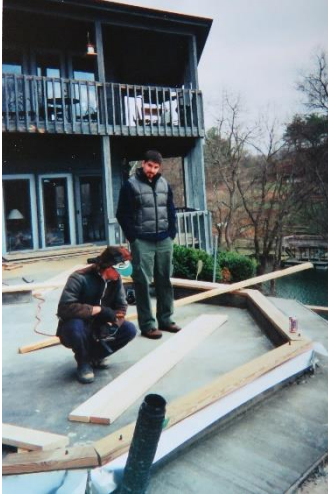
Foundation & a Sidewalk Superintendent
