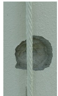
Closeup of west side of lighthouse
